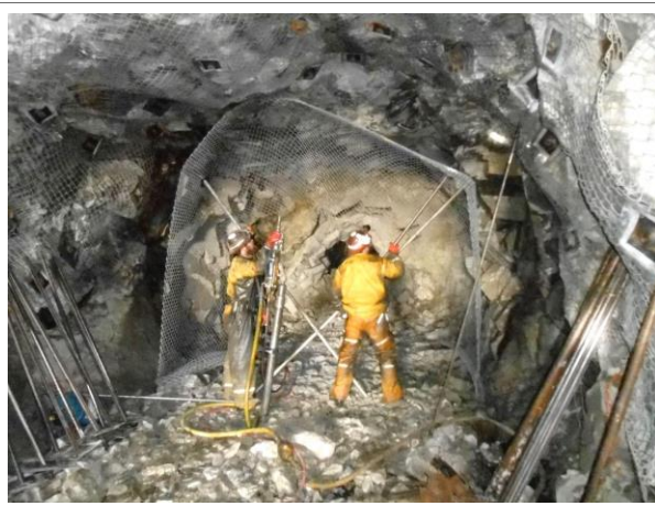
Installing Rock Bolts at South Mountain Mine
